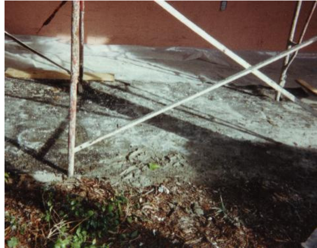
Figure 12. Scaffolding and mud sills
