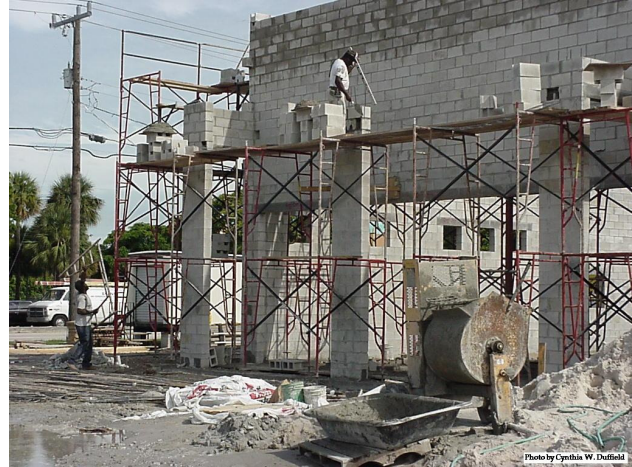
Figure 13. Scaffolding erected at a construction site
