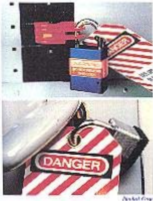
Figure 10. Equipment must be locked out and tagged out before preventive maintenance or servicing is performed.
