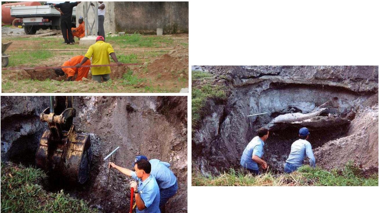
Figure 15. Examples of trenches and excavations.
